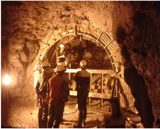
Photograph 3 Treatment of Cavity Zone
