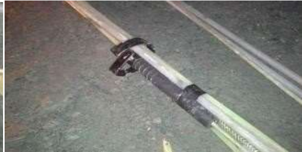
Figure 4b Rods with PVC Pipe
