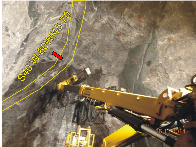
Figure 3 Joint 240-260°/65-70° exposed at chainage 113 m during pilot tunnel excavation
