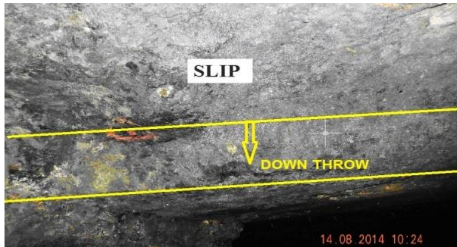
Picture 2 Minor Slip with Down Throw in Dip Gallery
